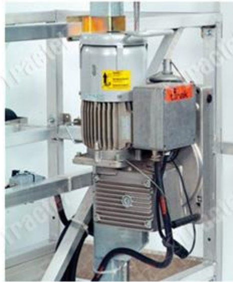
X-type installed on a working platform
